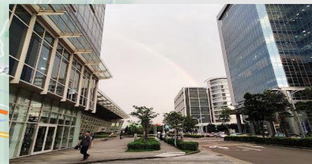
Tai Yuen Hi-Tech Industrial Park Office
